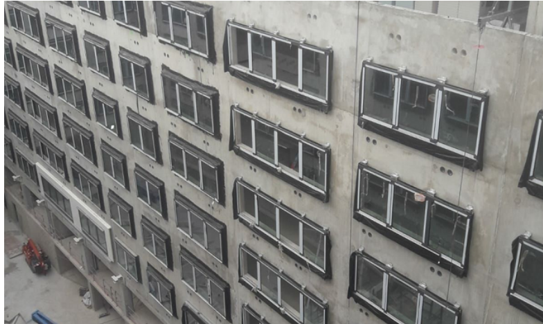
Image 1 - EPDM Membrane applied between window and concrete wall
