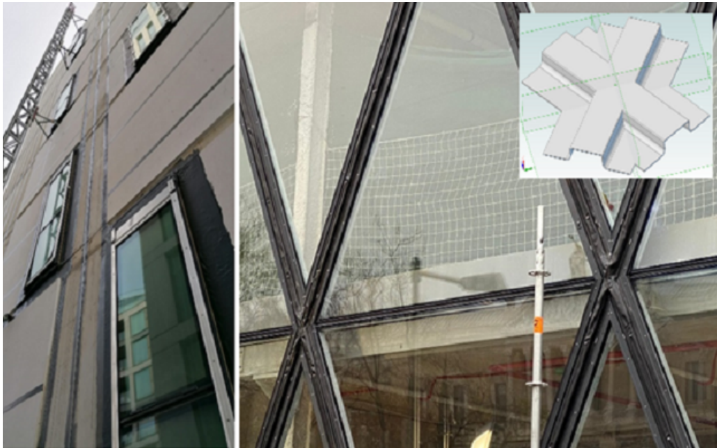
Image 5 - EPDM Façade Applications
