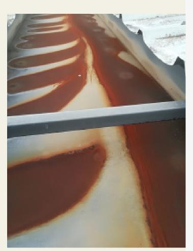
Failures in any system will always become evident at its weakest point, which in a gutter system is going to be the joints and changes of direction. Once corrosion has set in and a joint has started to fail, building movement, thermal expansion, freeze/thaw will further exasperate the problem. Once a joint has opened up it can be difficult to fix because of the build-up of dirt, debris and moisture around the opening.
