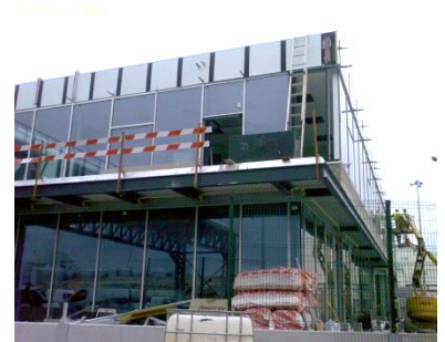
Sealing facade joints
