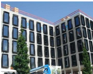
Sealing windows' frameworks
