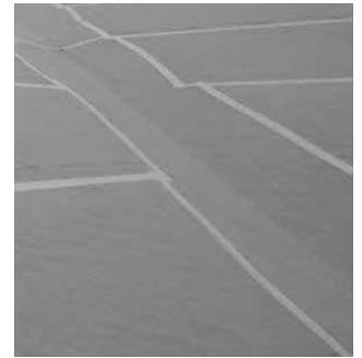
7. Sealing overlaps on vapour barriers
