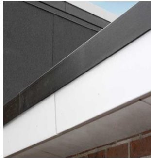
2. Sealing joints in roof edges/curbs
