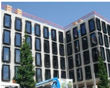
Sealing windows' frameworks
