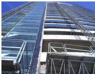
Sealing facade connections' perimeters
