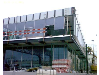
Sealing facade joints
