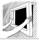
When placing the frame, pressure must be developed on the aperture lower side and the frame should be fitted and leveled within the opening. Any movement of the Effisus SealExpand Tape occurred during or after the frame placement can be corrected using a spatula. When positioning shims pay special attention so it does not overlap the tape bonding area. If there is any esthetical demand, the tape can be painted or covered with sealant after being installed.
