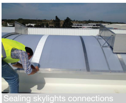
Sealing joints in metal roofs
