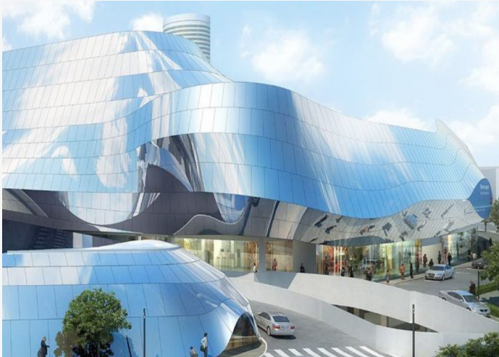
Birmingham Station Project, (United Kingdom)
