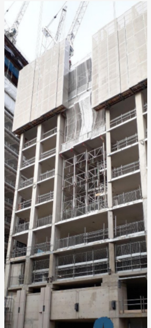
Facade Precast Panel Assembly
