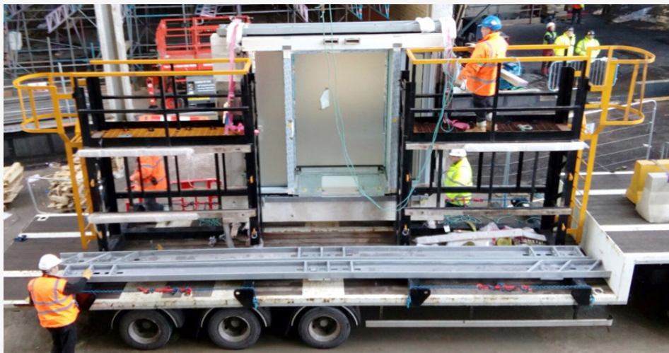
Transportation Pre-fabricated Precast Panel
