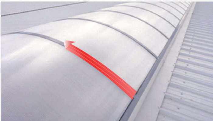
1 – Sealing joints on polycarbonate curve skylights
