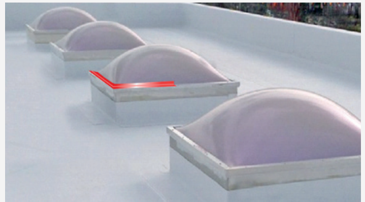
2 – Sealing joints between metal flashing and polycarbonate skylights
