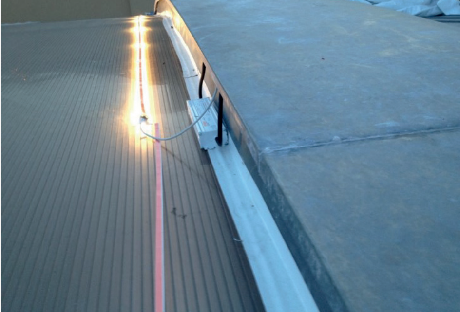
1 – Hotel – Joints between polycarbonate and metal
