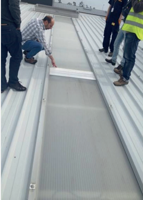
1 – Industrial building – Joints between polycarbonate panels
