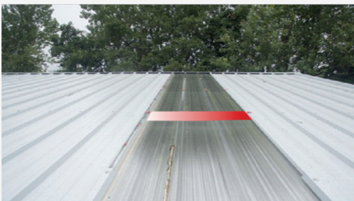
3 – Sealing joints between polycarbonate sheets and corrugated metal roofs
