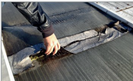
Typical pathologies on joints of polycarbonate structures
